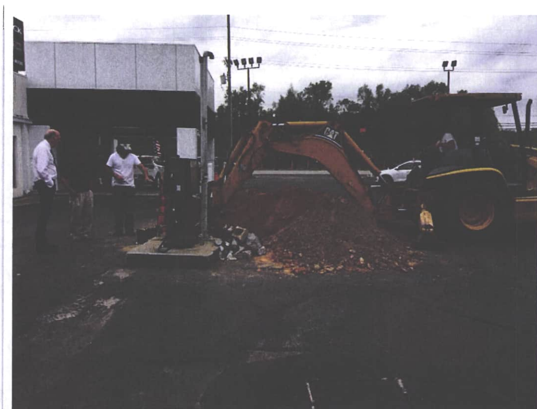
Initial UST Excavation with Backhoe
