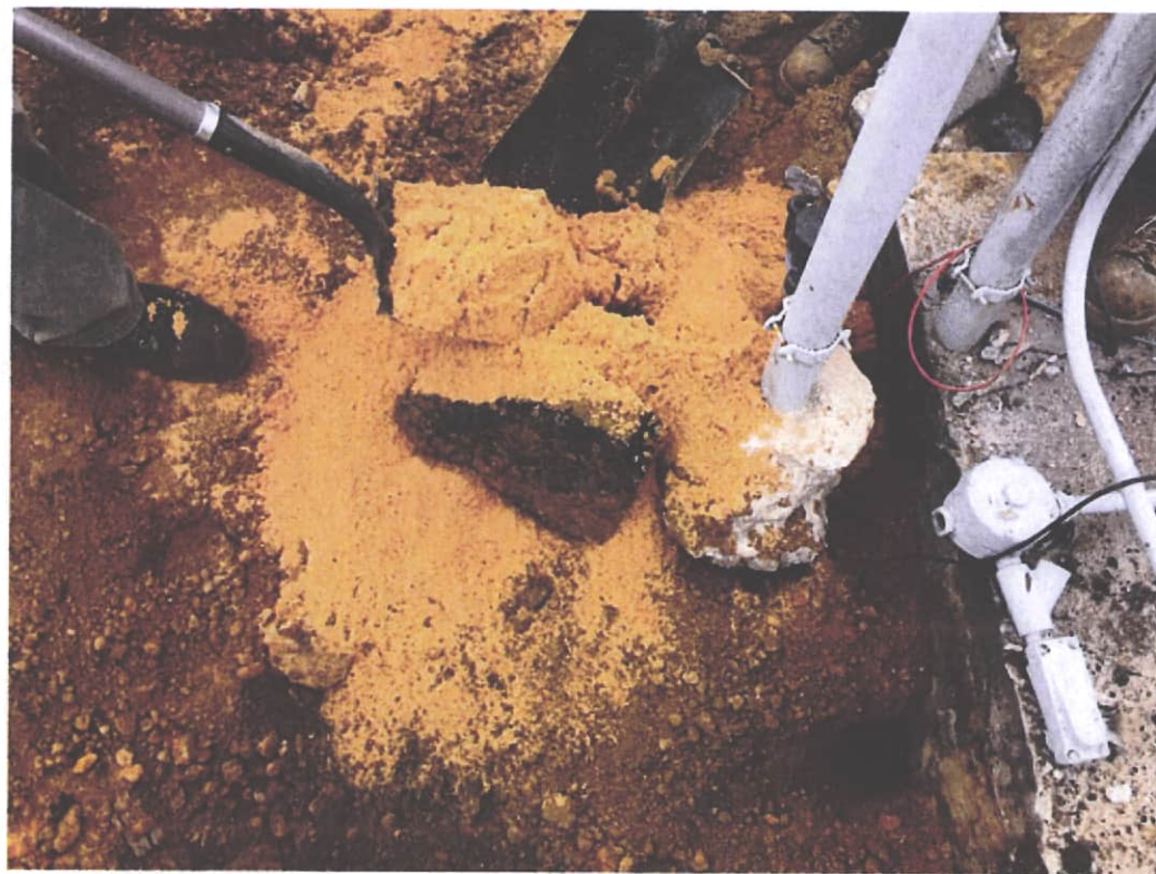
Manually Filling the UST with Sand
