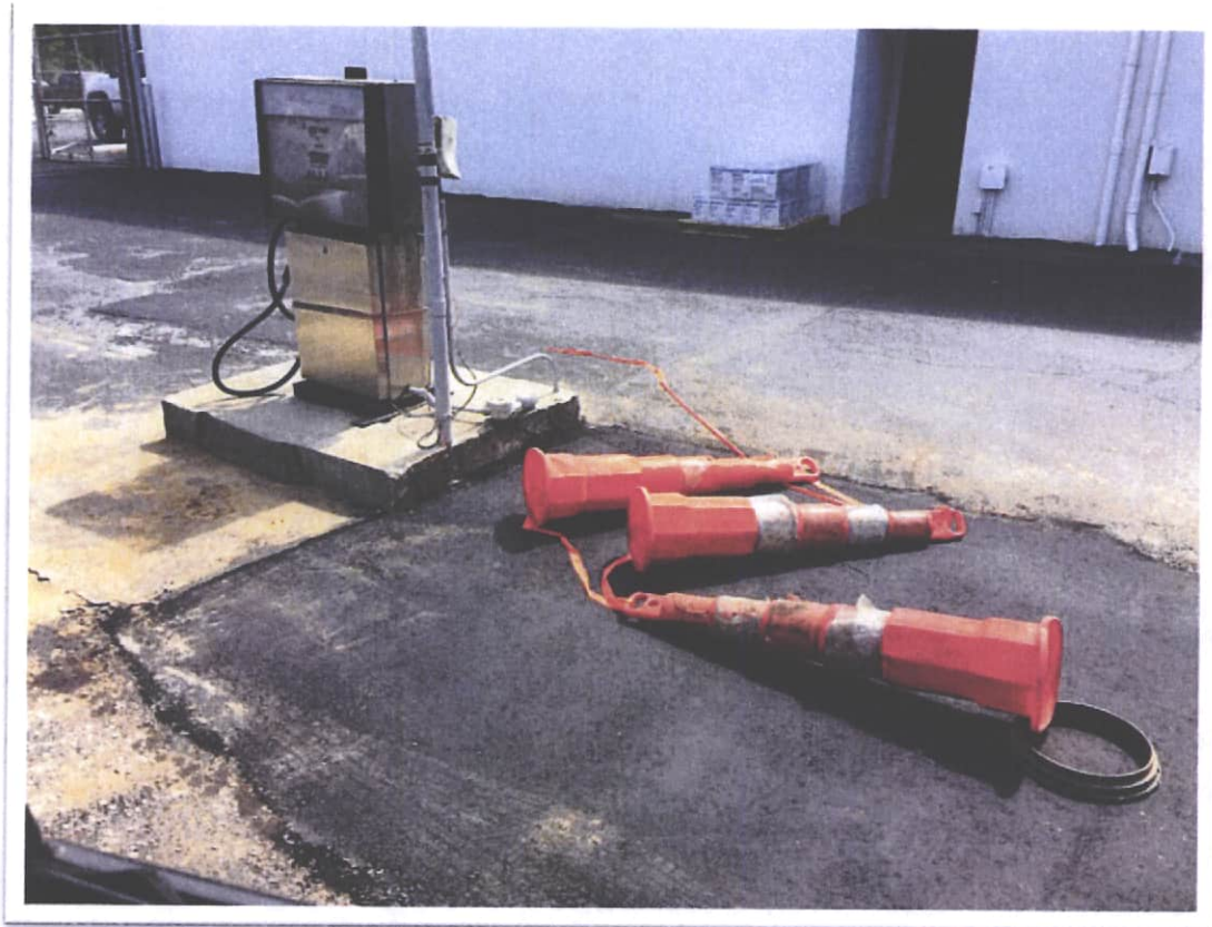
Asphalt Patch above Abandoned UST
