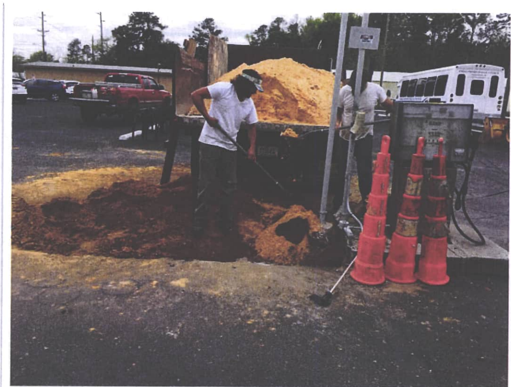
Unloading Sand for UST Abandonment
