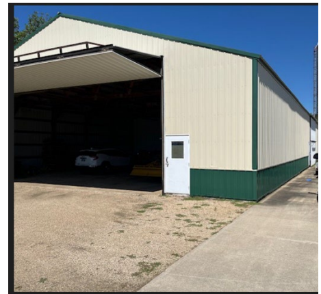
(showing hydrolift door)
