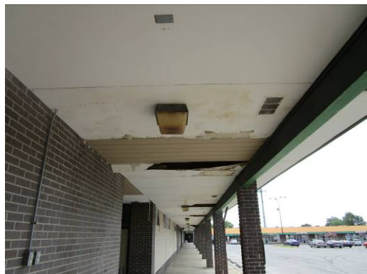
6. Typical soffit damage.
