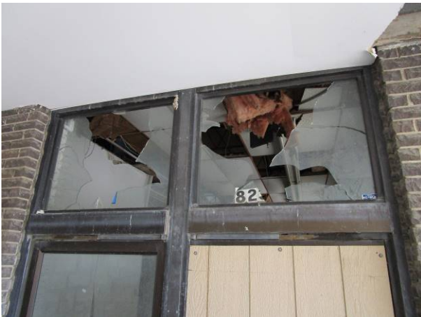
1. Example of damaged windows
