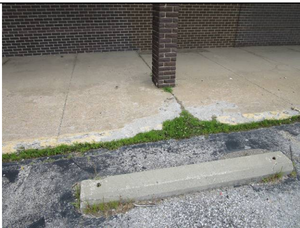
1. Example of damaged walkway
