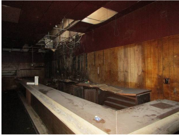
3. Example of damaged interior finishes
