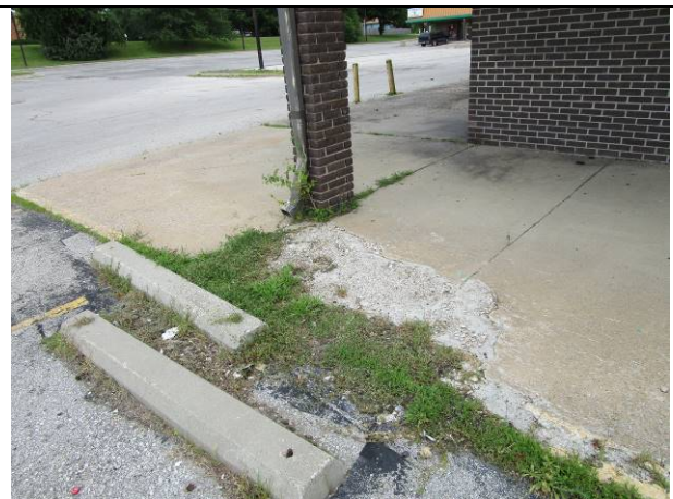
2. Example of damaged walkway
