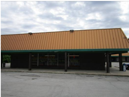
9. Typical soffit roof configuration.
