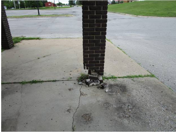
1. Example of damaged pillar
