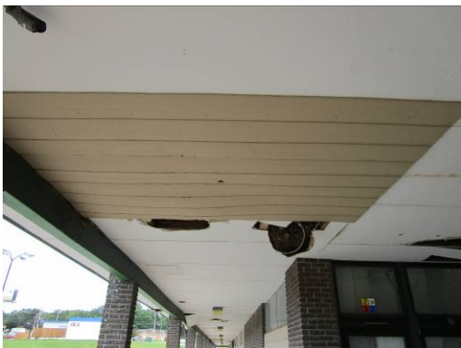
5. Typical soffit damage.
