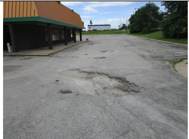
2. Example of damaged parking lot
