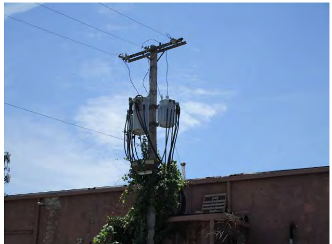
12. Typical pole mounted transformer
