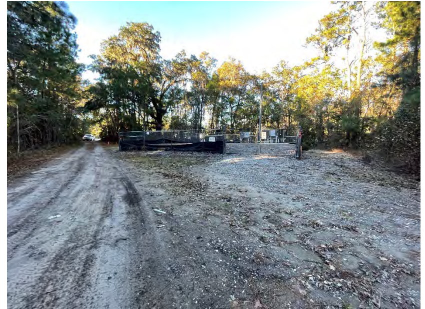
Photograph 28. A lift station located on the adjacent property to the northwest.
